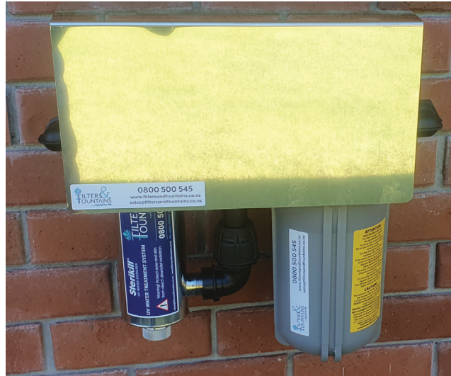
Single UV Steriliser unit - with cover (above), and (below) without cover.
