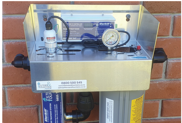
Single UV Steriliser unit - with cover (above), and (below) without cover.
